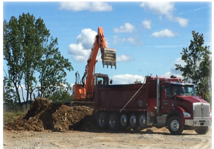
Impacted Soil Remediation
